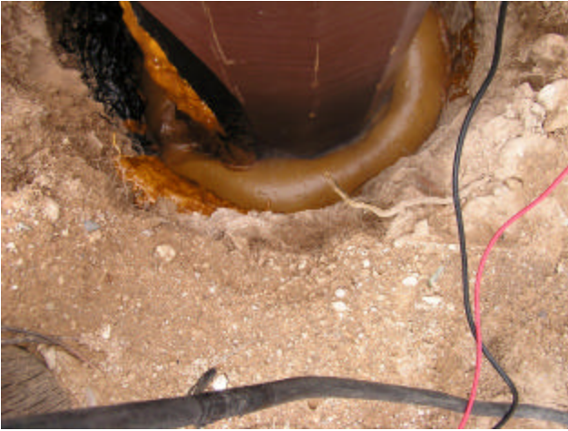
Photo Showing Finished Structure with Megger Wires attached
