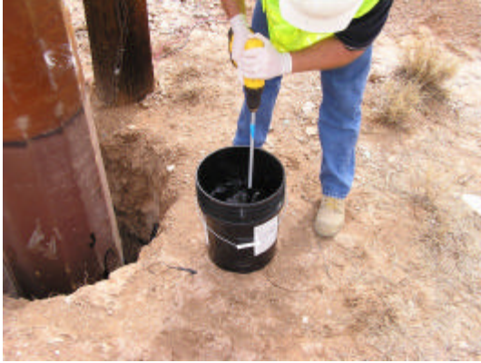
Poly-Ground Being Mixed On-Site
