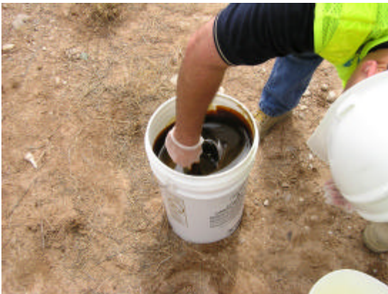
Photo Showing Poly-Set Being Hand Mixed
