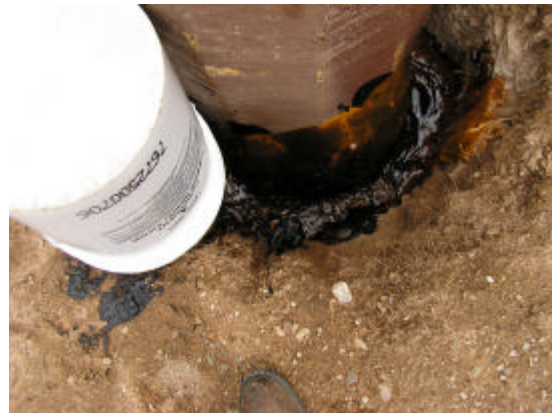
Photo Showing Poly-Set Being Poured Into Hole
