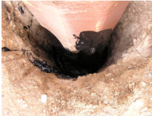
Finished Poly-Ground Portion
