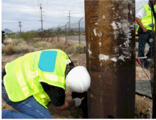
Poly-Ground Being Poured Into Hole
