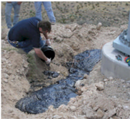
Pole 4: This photo shows the “connecting” of the two plates using a Poly-Ground® only connection and the subsequent reading, keeping in mind there is still only a bottom connection to the earth.
