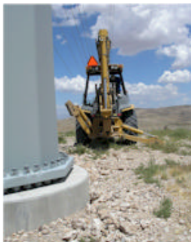
Pole 4: This structure was set on a pre-cast concrete foundation that had a galvanized plate put in the trench but was not treated with any backfill other than native earth. The plate was placed vertically in the trench and backfilled with the excavated material. The reading was 98.0 ohms.
