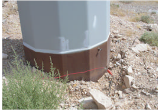
Pole 3: This particular pole had been post-installation retro-fitted with the above described steel plate backfilled with Poly-Ground ® . It also had a driven rod that was installed during the initial installation.
