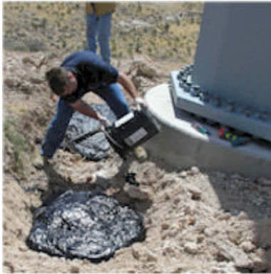
Pole 4: This photo shows the second installation and megger reading was 103.4 ohms. This reading is a cumulative reading of the first plate tied together with the second plate. So there are actually two plates tied together being read here, but there is still only bottom contact being made as the hole is still open air.
