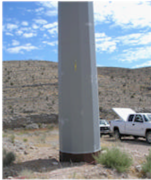
Pole 3: This particular pole had been post-installation retro-fitted with the above described steel plate backfilled with Poly-Ground ® . It also had a driven rod that was installed during the initial installation.
