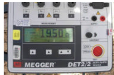
Pole 1: This is a close up view of the actual reading obtained on the above structure. The two red leads are attached to the grounding electrode itself, and the yellow lead is attached to a stake at 62' from the electrode and the blue is attached to a driven stake at 100'. The resistance reading was 19.50 ohms.
