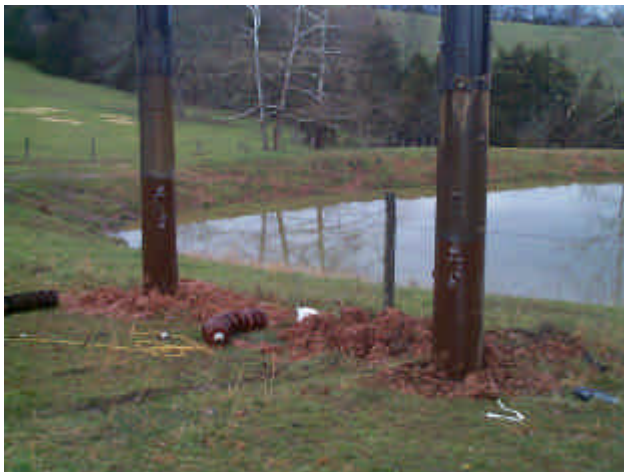
Photo showing finished structure
