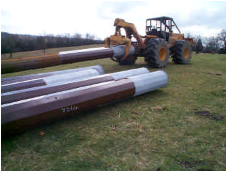
Photo showing poles prior to installation
