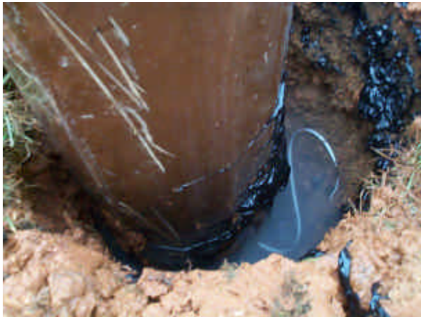
Photo showing Poly-Ground installed prior to Poly-Set backfilling
