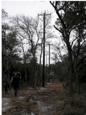
Photo showing the remote location of the initial Poly-Set® installation.
