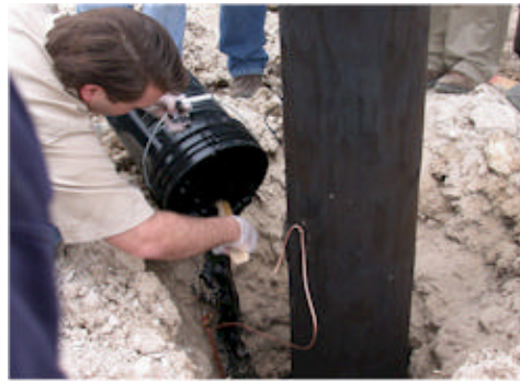
Photo of Poly-Ground being poured
