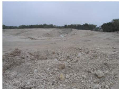
Below: Photo showing another view of the jobsite.
