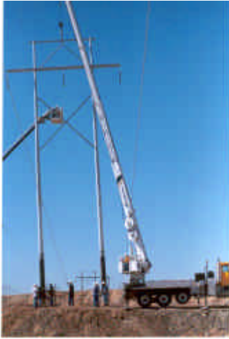
Pole being lifted into position
