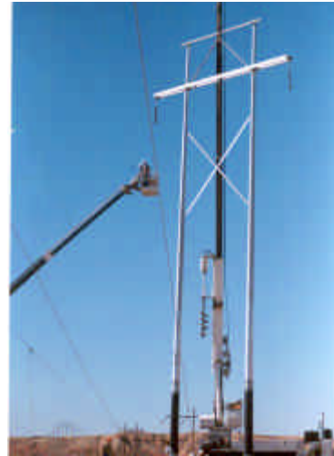
H-Frame being set into position
