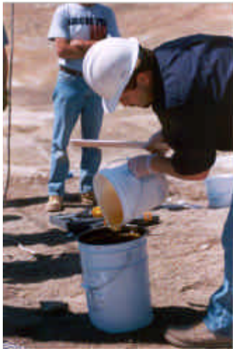
Mixing materials on the job site
