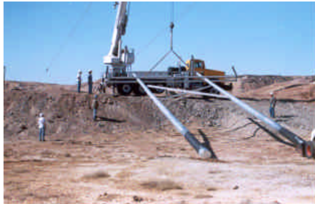
H-Frame on the ground being lifted
